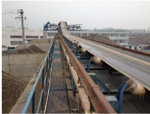
Gambar 35. Coal Handling Unit
