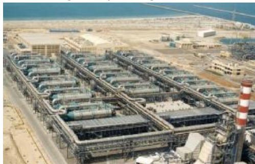
Gambar 32. Desalination Plant (Sumber: Utilities Middle East)
