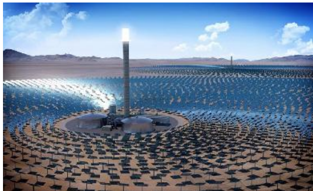
Gambar 78. Concentrated Solar Panel (Sumber: Heliocsp)
